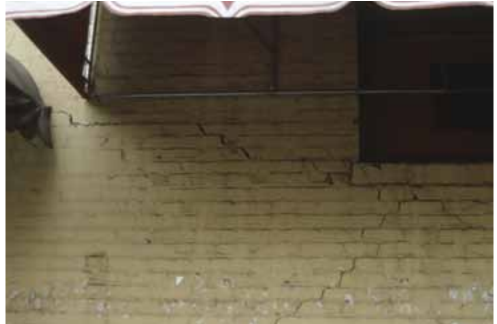
Above: Cracks in wall of building on Broadway, October 20th 1989. A few more seconds of shaking and this building would probably have been red-tagged. (Photo by M. Collier)
